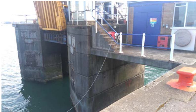
Figure 2.6 Existing Seaward Edge of Buffer Dolphin Showing Forward End of Linkspan Ramp
