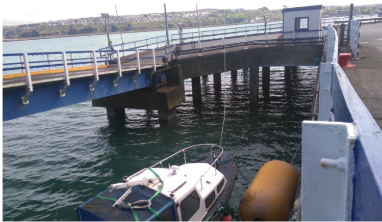
Figure 2.3 Existing Open Piled Deck, Bankseat and Linkspan Ramp
