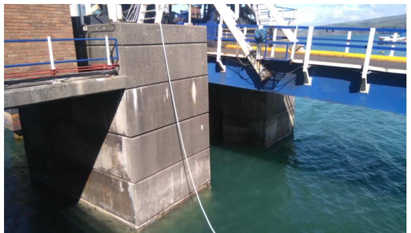
Figure 2.5 Existing Landside of Buffer Dolphin and Linkspan Ramp
