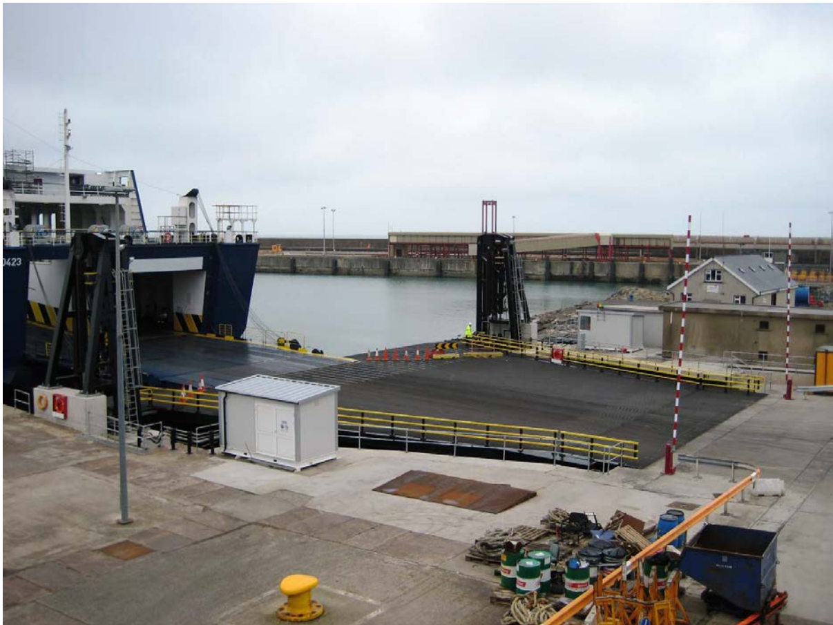
Figure 2.11 Typical linkspan
