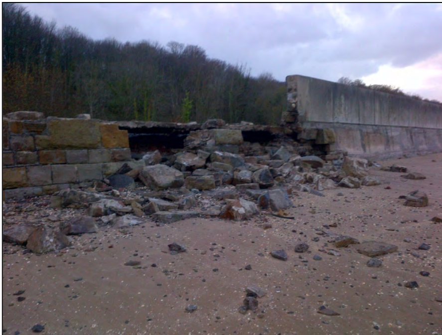
Network Rail Damage
