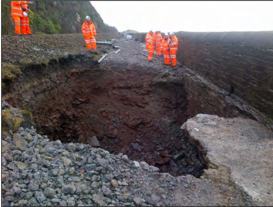
Network Rail Damage
