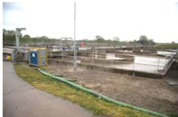
Natural Resources Wales, Dee River Basin District Five Fords waste water treatment plant
