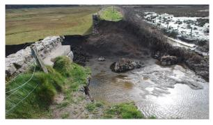
Agreement has been reached with Swansea City Council, the local ramblers group and the local community on a solution to the loss of the path over the breached sea-wall at Cwm Ivy. The plan is to widen the breach and create a culvert-causeway which will allow the tide to continue to flood the marsh, and enable the saltmarsh restoration project to continue.
