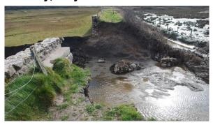
Agreement has been reached with Swansea City Council, the local ramblers group and the local community on a solution to the loss of the path over the breached sea-wall at Cwm Ivy. The plan is to widen the breach and create a culvert-causeway which will allow the tide to continue to flood the marsh, and enable the saltmarsh restoration project to continue.
