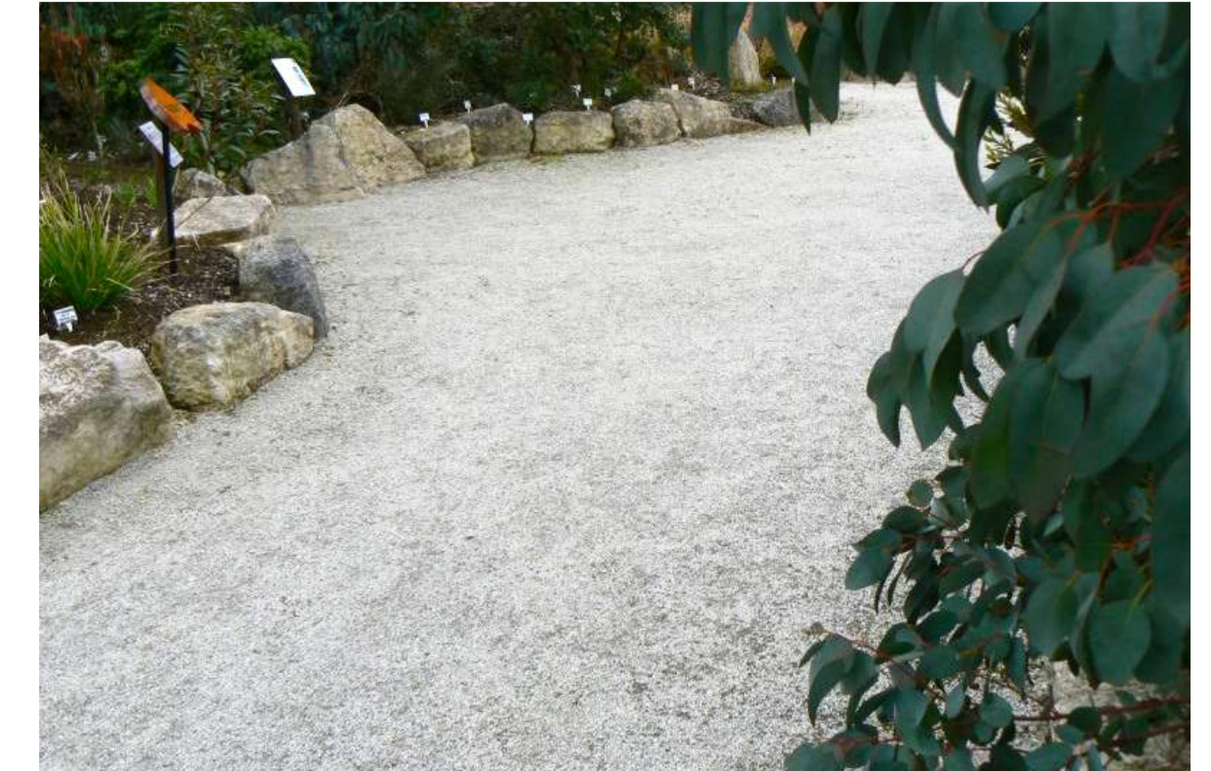
Llwybr malurion cerrig nodweddiadol Crushed stone self-bound path
