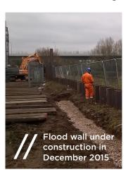
The works involved the construction of a 150m long floodwall along the Rhymney River embankment, off Newport Road in south Cardiff. Our contractor GBV, completed the works in December 2014. The floodwall directly improves the standard of protection to 12 local businesses in the Rhymney River Bridge Road Industrial Estate and, when later phases of the flood scheme are constructed, the wider Newport Road/Colchester Avenue area.
