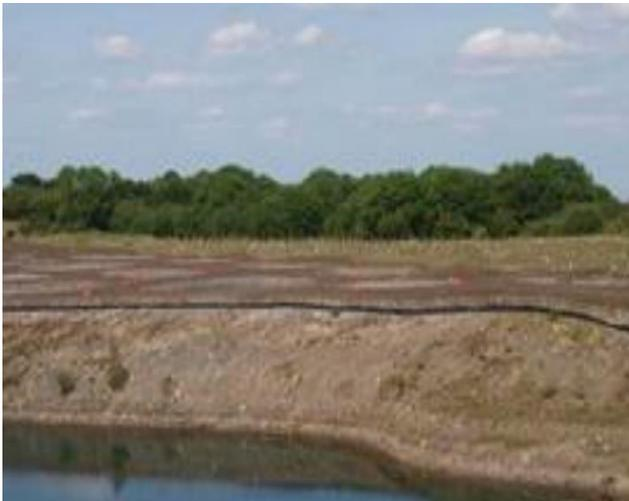
The land was originally an abandoned claypit with an unsafe steep-sided lagoon. This lagoon had to be filled in to create open space for the new properties and over 50 ponds were also created as part of the new habitat.
