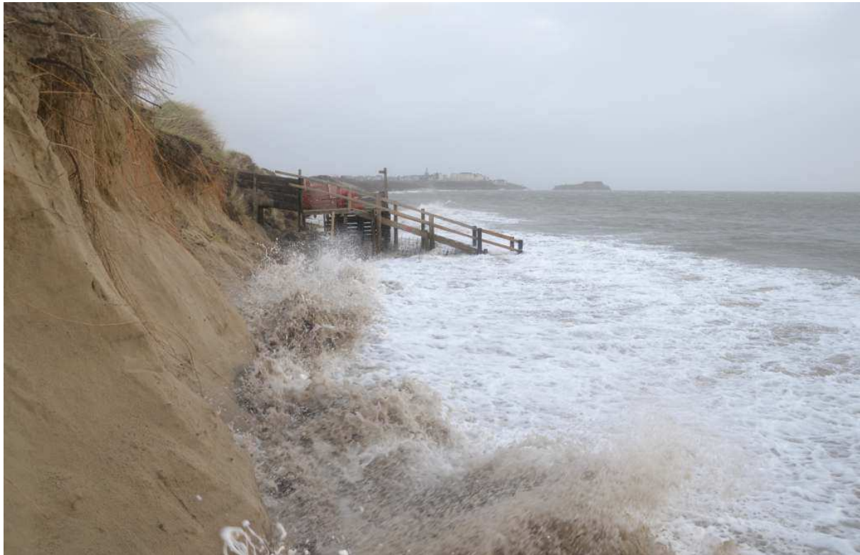
Figure 5. Erosion of the dunes in action at Penally on 6th January 2014 (Sid Howells, Natural Resources Wales).
