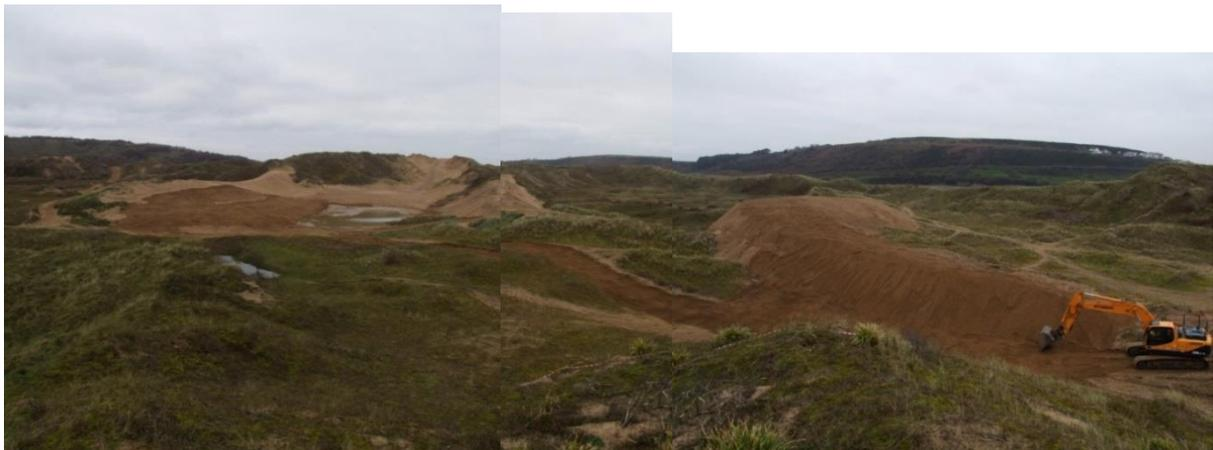
**Figure 33.** Merthyr Mawr Phase 2 area. View of work area looking east at end of contract, with area of sand excavation on the left and artificially constructed dune on the right (photograph by D. Ludlow, NRW)
