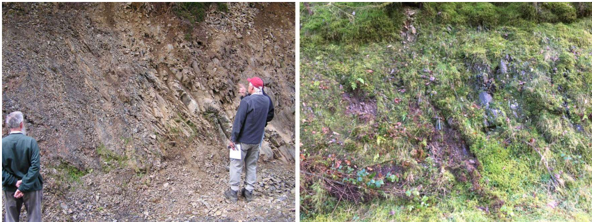
Figure 5. Base of Bronydd Formation, Scrach Track GCR site. Following clearance of the site in 2009 (left hand image) and as it is now (March 2019) (right hand image) with hammer showing approximate location of contact
