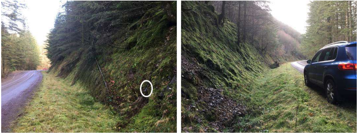
Figure 8. General views of the Scrach Track GCR site to the east (left) and west (right) of the Garth House Formation and Bronydd Formation contact (circled hammer) showing the current overgrown state of the section
