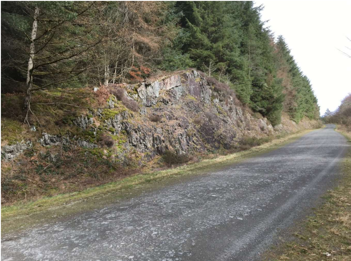
Figure 11. Coed-cwm-Aeron Track GCR site. The weather-resistant nature of the Cefngarreg Sandstone Formation that occupies the bulk of the track cutting is reflected in the better condition of this site, which currently requires little remedial work (see text)
