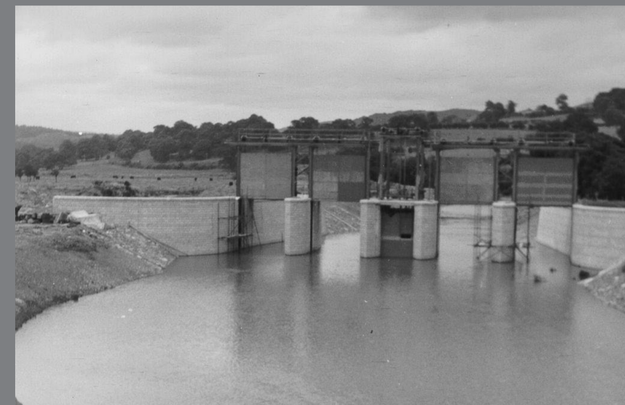
Adeiladu'r llifffordau Sluices during construction
